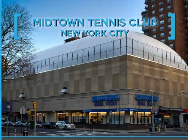
Arizon designed an air-supported building that fits seamlessly into the fenced-in tennis area on the roof of a building in Manhattan. The dome is installed annually in early fall and dismantled each spring. Arizon's design simplified the installation of the dome, despite seemingly difficult site conditions.
