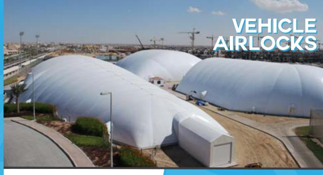
Large equipment, vehicles and trucks can be safely brought into an air-supported buildings by the use of a vehicle airlock system. Two large overhead doors at each end of an air-tight, fabric cooridor are coordinated so that only one high-strength automatic door may be open at a time, as to not compromize the dome's internal pressure.
