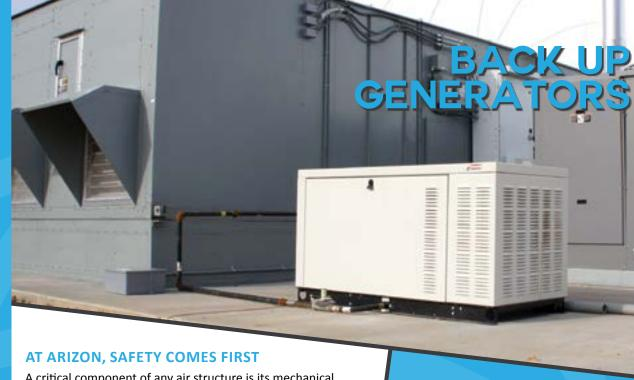
A critical component of any air structure is its mechanical operating system, which provides the pressurization necessary to keep the dome inflated. Arizon's air structure mechanical systems include emergency and back-up generators, in case the primary or auxiliary inflation systems have technical trouble or in case there is a power failure.
